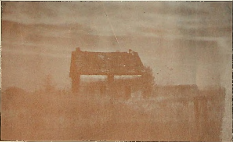
The only original building left on the townsite of Nantasket.
