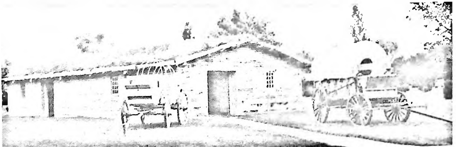
Reconstructed Blacksmith-Carpenter Shop with prairie schooners.
