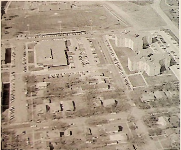
Arial image of where the shooting occurred. Nebraska Food Center building is under the football field. Newman Center is at bottom left of the photo.
