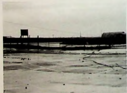
Damage at Baldwin's-down power lines Photo property of Todd Pickering, used with permission
