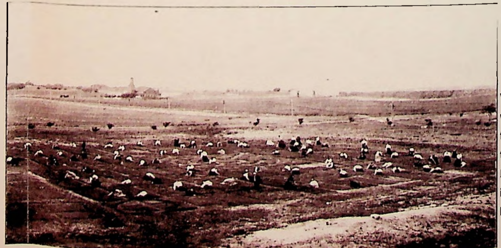
Women working in a field with the Kearney Power Plant in the background
